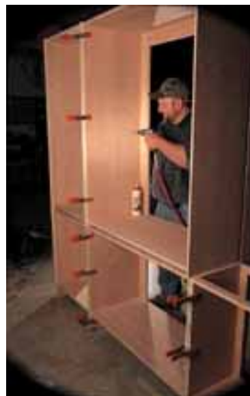
3 Then use spring clamps at the back to hold everything together as you screw the upper cabinets together and the lower cabinets together. Be sure to screw right behind the face frame so the screw is less visible.
